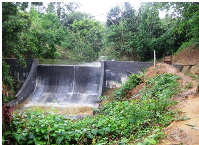
R.C.C. Dam and C.C.Irrigation Channel across Chiso stream at ChisoGaning under ChisoGaning River Valley Project (AIBP)
