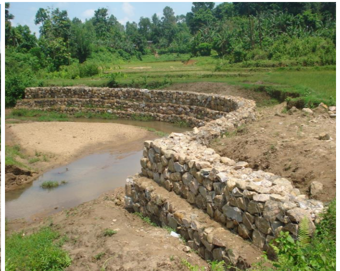
Boulder Sausage Protection wall along Chame stream of existing Paddy Field at Chame Watershed under AIBP, East Garo Hills, Songsak Block
