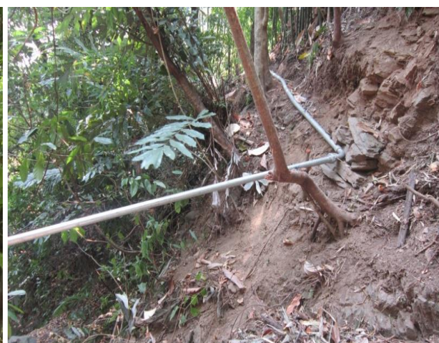
Bamboo channels replaced by GI pipe line
