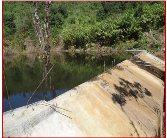
UPSTREAM VIEW OF THE CHECK DAM AT MAWPRAN RWH UNDER RKVY 2010-11
