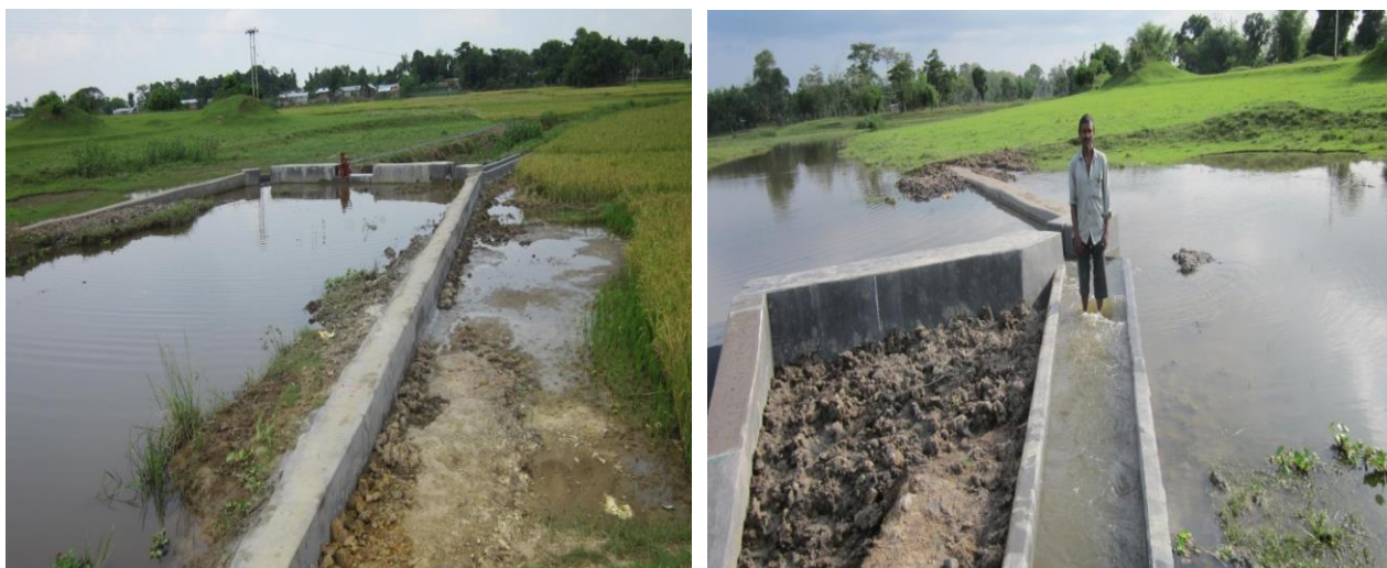
PUCCA CHECK DAM AT HARIBANGA
