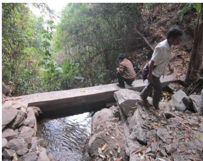
Check dam/head dam at the source (intake point)
