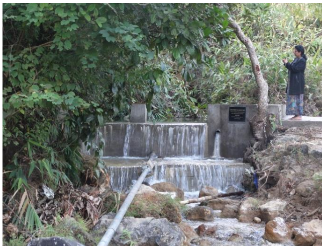
Sluice Gate at Rajai
