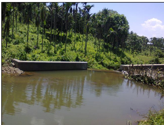
A View of the Irrigation Check Dam
