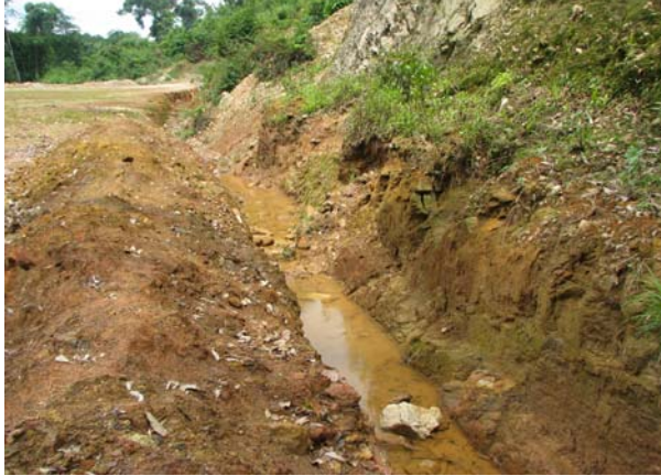
Drain - South side
