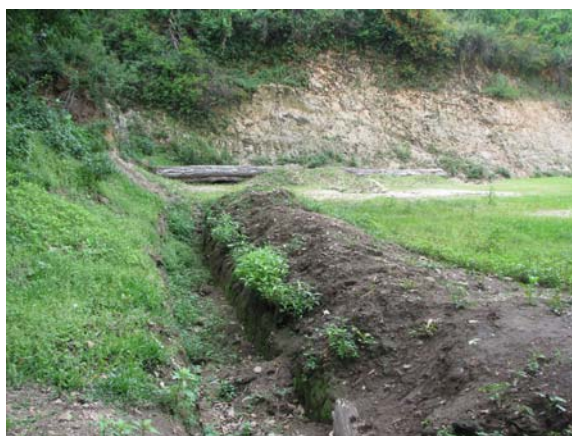
Drain – West side
