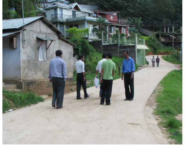
Motorable road (cement)
