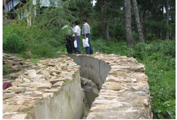
Drain cum motor-able road
