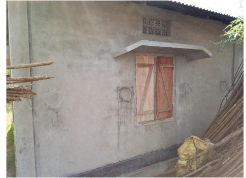
Completed IAY House
