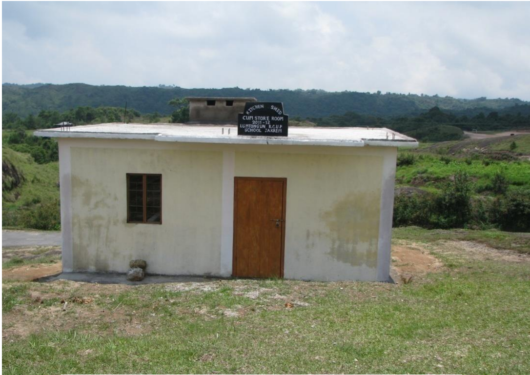
Kitchen shed cum store room under Mid Day Meal Scheme.
