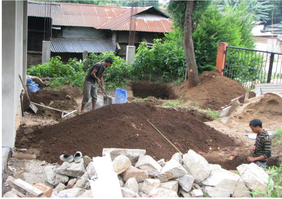
Work for construction of Kitchen shed in progress.
