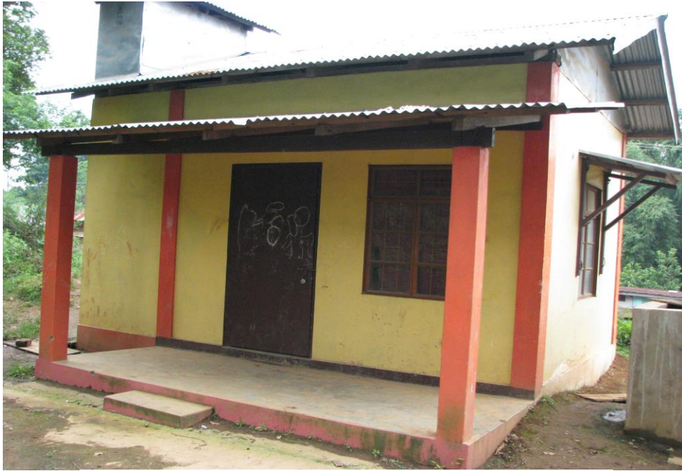
Kitchen shed constructed under Mid Day Meal.
