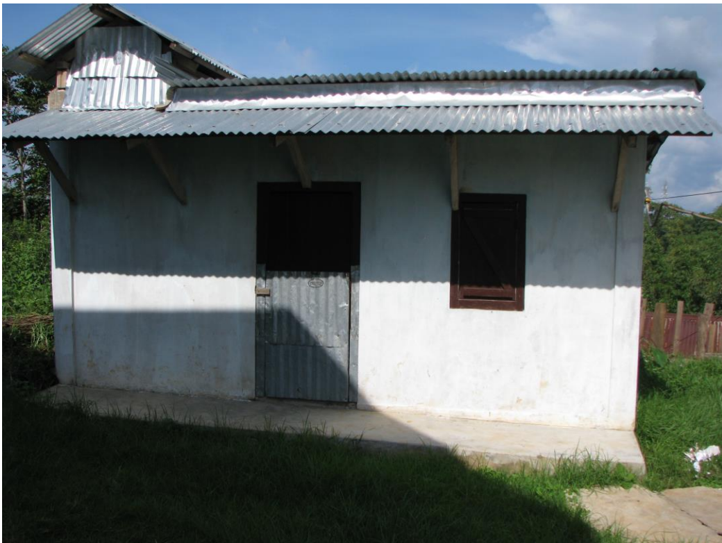
Kitchen sheds constructed under Mid Day Meal.
