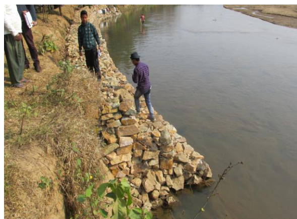
Boulder Sausage under construction
