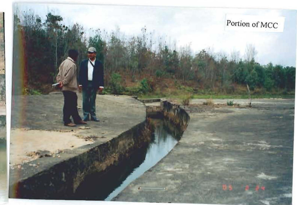
Big leakage of water from the left wall/platform
