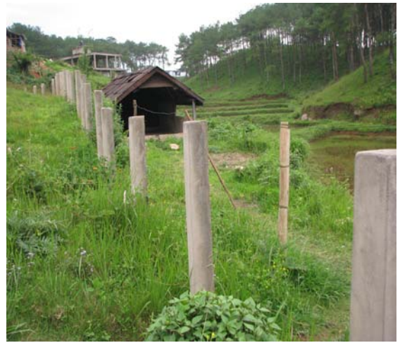
Part of fencing – Cement pillars
