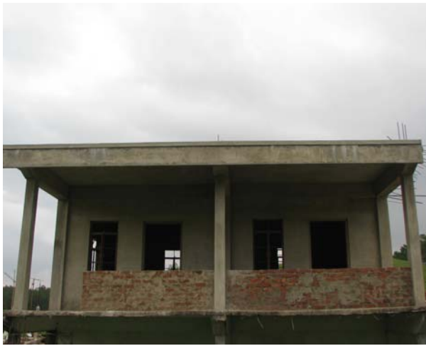
Classroom under construction – 1 st Floor
