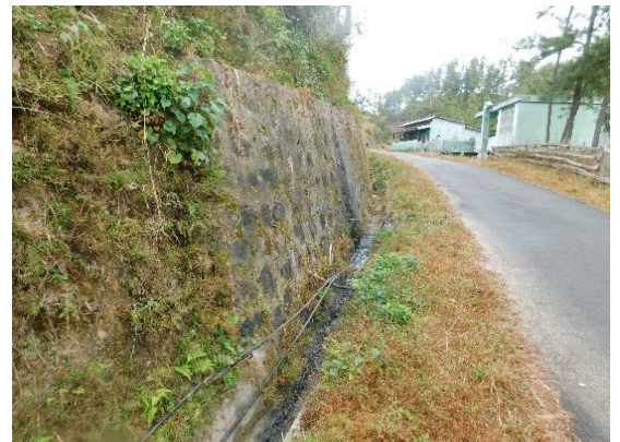
Retaining Wall
