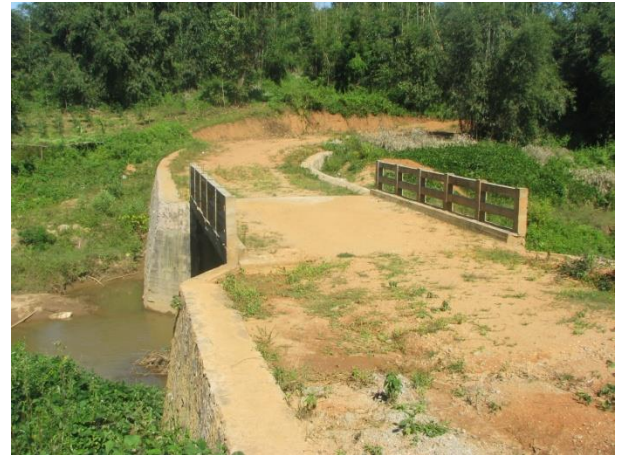
RCC Bridge and Retaining Wall
