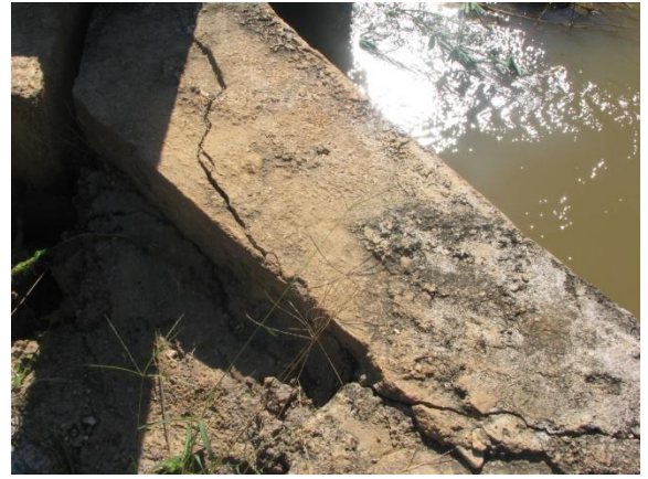
Crack on Wing Wall of a Bridge
