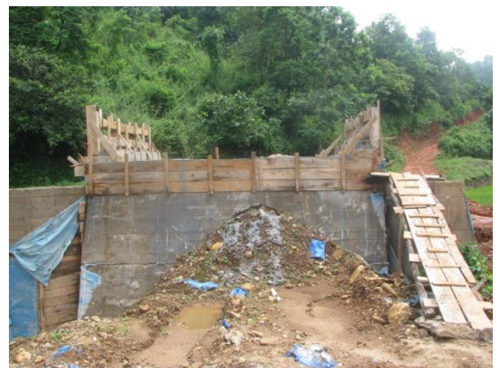
RCC Bridge under construction
